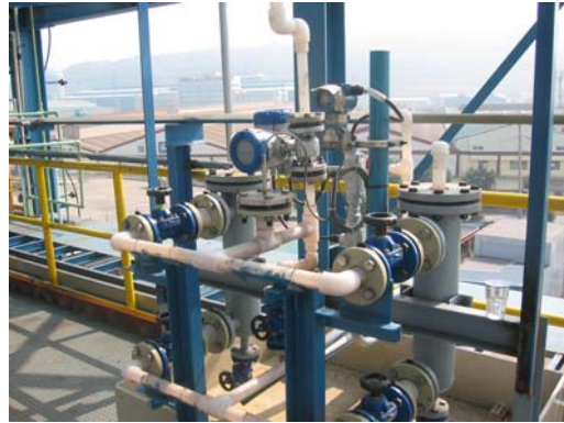
OPTIFLUX 4300 with virtual reference at Andritz
