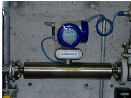
OPTIMASS 7300 C Tantalum doses highly aggressive liquid
