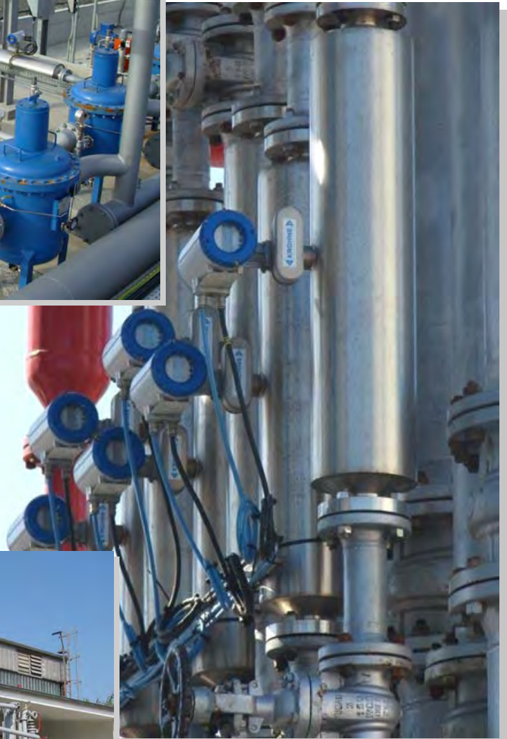
Top: Meters installed in a Custody Transfer application. Note the air eliminators upstream of the flow meters.
