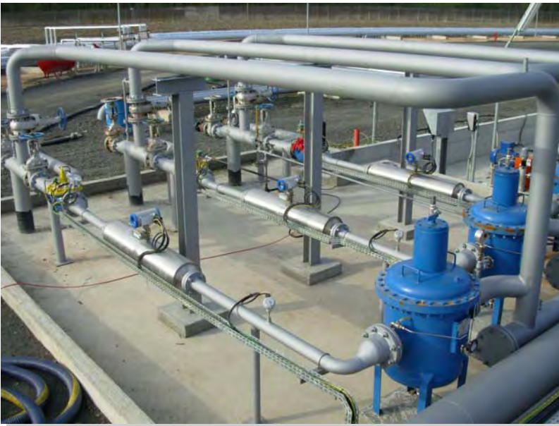
Top: Meters installed in a Custody Transfer application. Note the air eliminators upstream of the flow meters.
